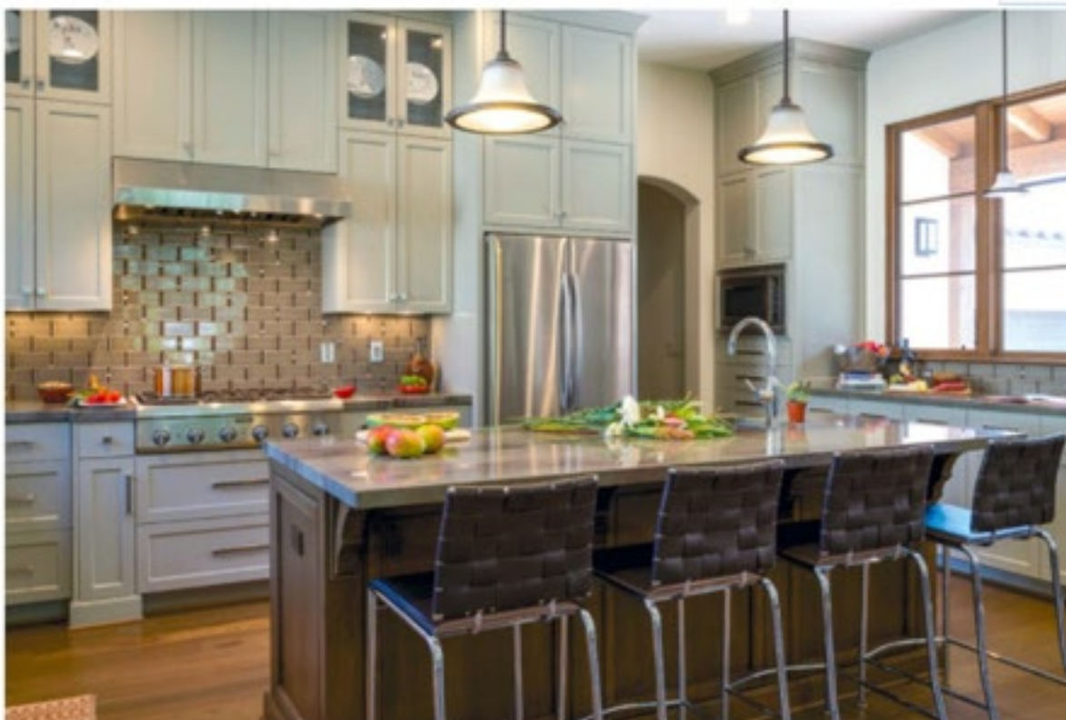
For this subway tile backsplash, CTD inserted cranberry glass and chrome mosaic tiles intermittently throughout the brick-lay pattern so that the backsplash would highlight the colors in the island's counters.
